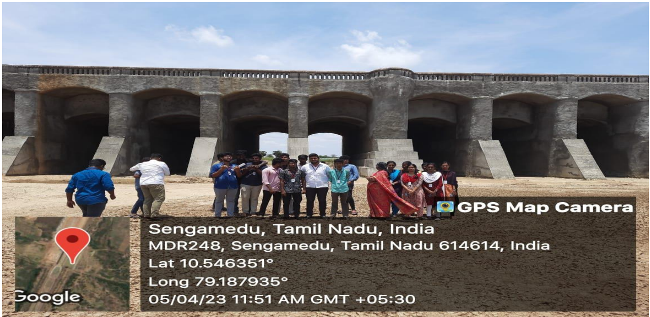
Cross drainage work-Aqueduct near Vettikadu
