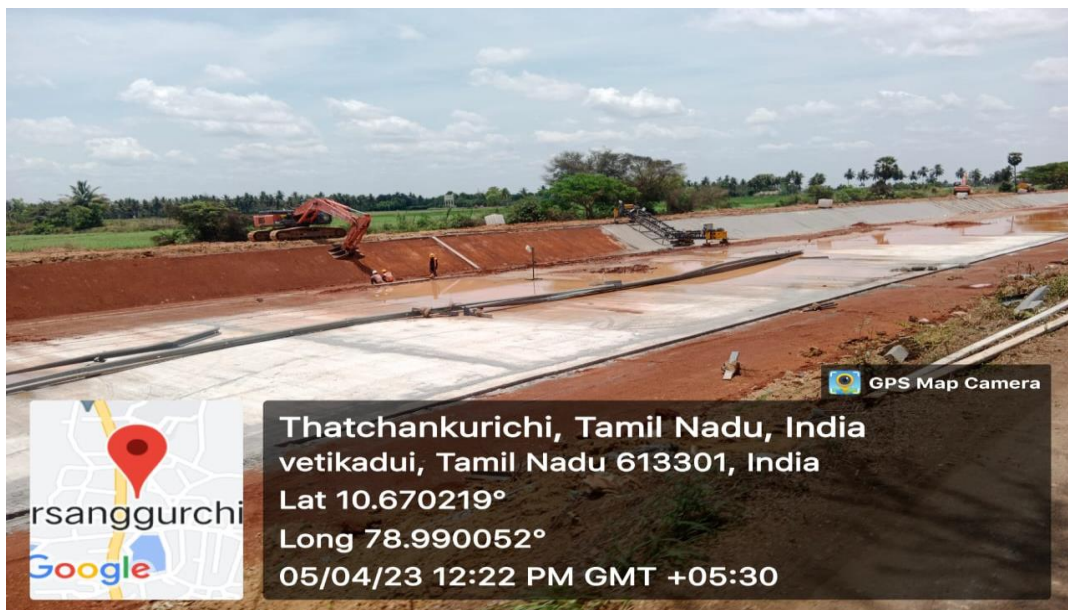
Lining of Canal- Near Vettikadu
